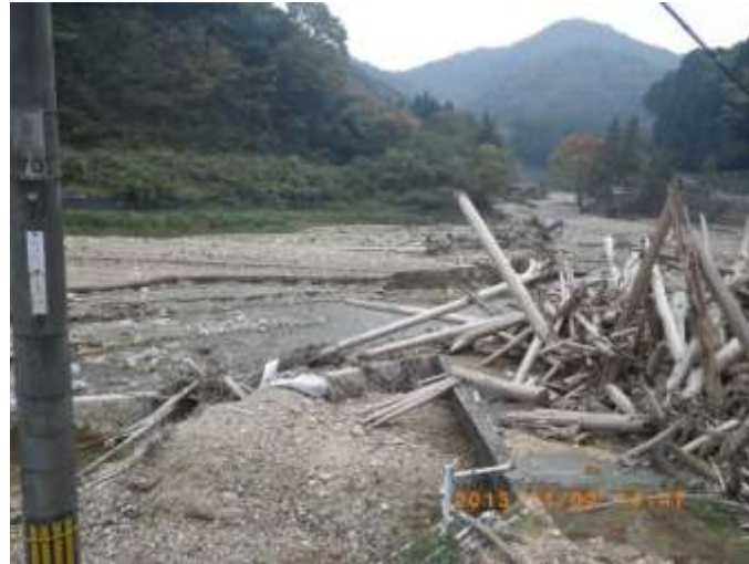
Figure 1. Woody debris accumulation at the bridge.
